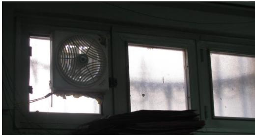
Figure 3. A small ventilation system with poor insulation in the building
