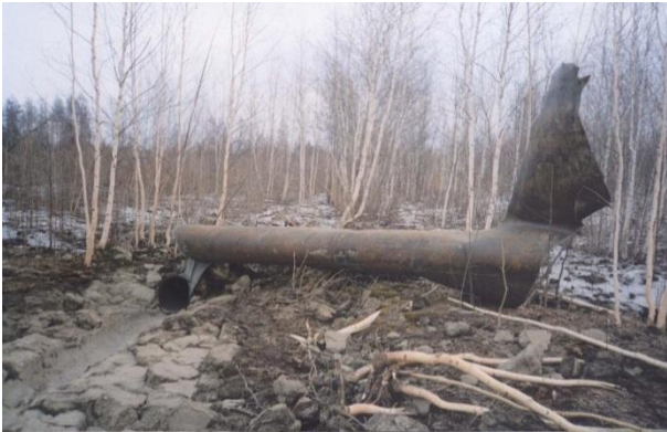
Figure 1. Fracture of the main gas pipeline
