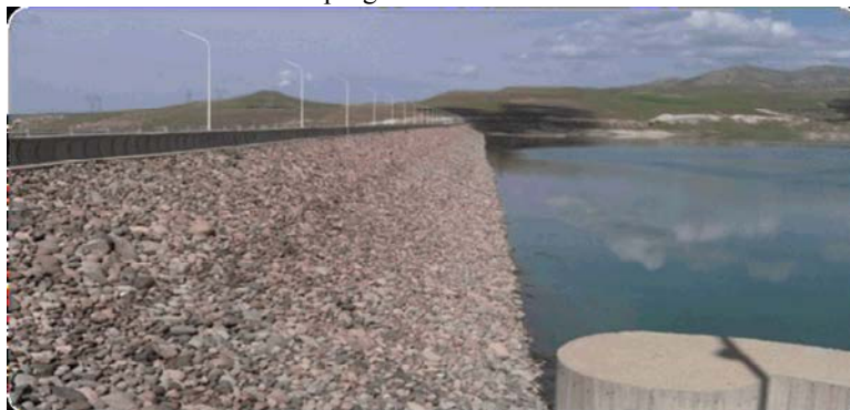
Fig. 1: Upstream slope of Alavian reservoir dam
