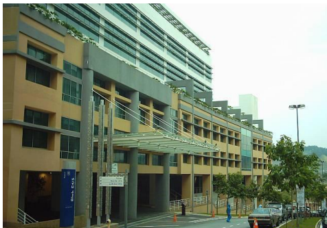
Fig. 2: a) Main entrance of the MEGTW building, Putrajaya
