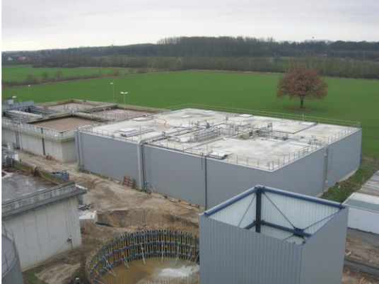
Figure 3. View of the PANDA plant at Rheda-Wiedenbrück during construction
