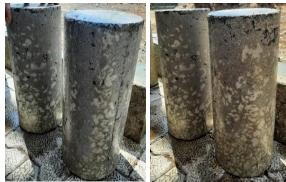
Figure 6. Map cracking on concrete
